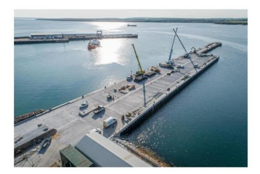
The current forecast completion date remains 8<sup>th</sup> October 2021. The final concrete pours and dredge surveys are scheduled for this week. The final construction activities include installation of cathodic protection, fenders, lighting masts, security fencing and toe rails.
